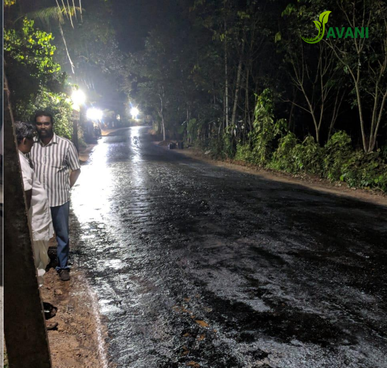
EMULSION COATING BEFORE ASPHALT
