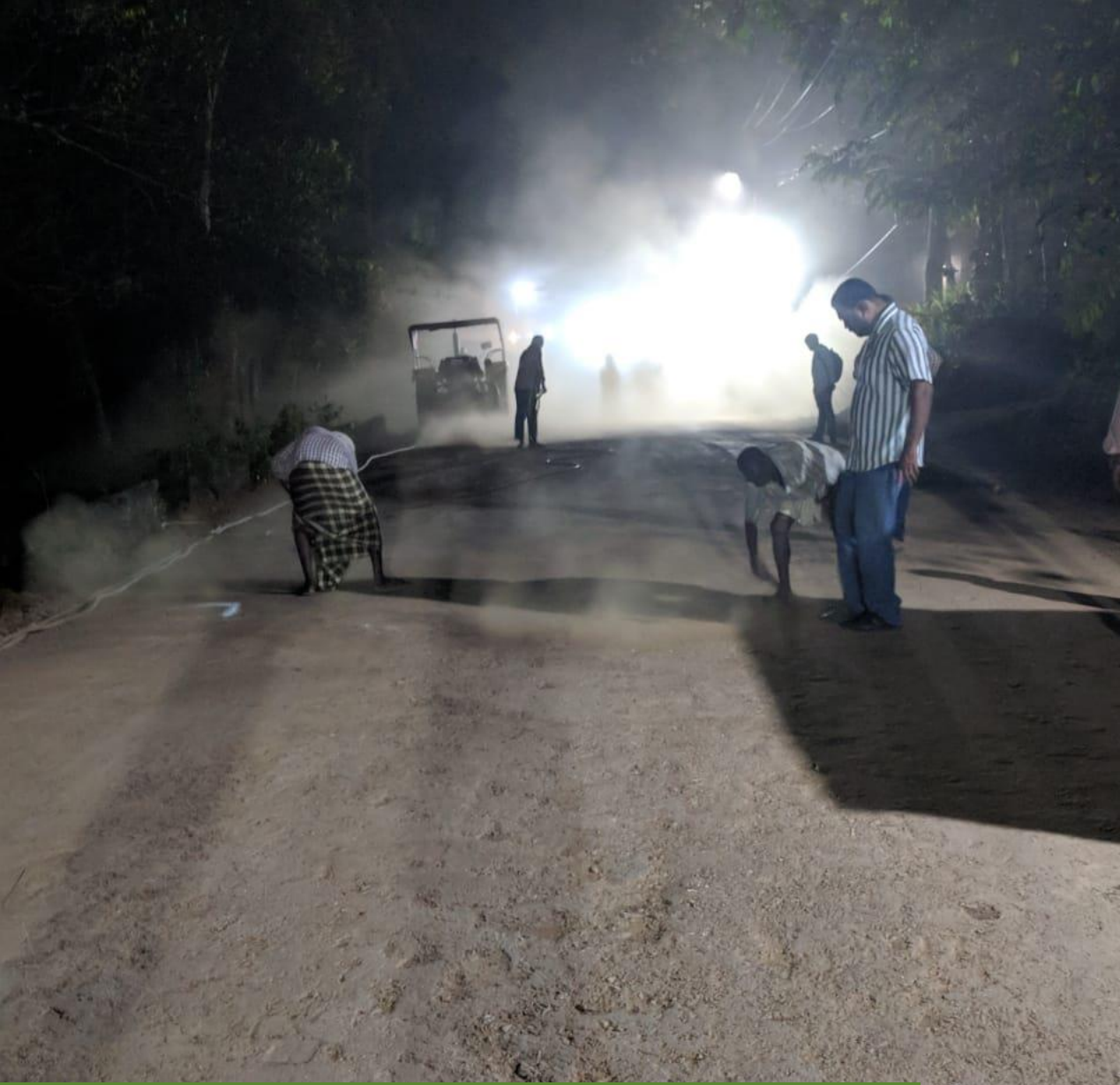
CLEANING OF SURFACE BEFORE EMULSION
