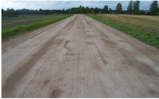
Picture 28. Gravel road stabilized with StabilRoad® and cement
