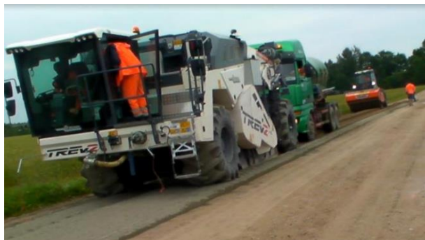
Picture 20. Soil stabilization with StabilRoad® and cement
