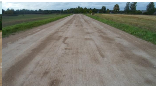
Picture 21. Surface after stabilization with StabilRoad® and cement
