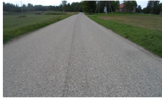
Picture 29. Gravel road stabilized with StabilRoad® and cement and coated after
